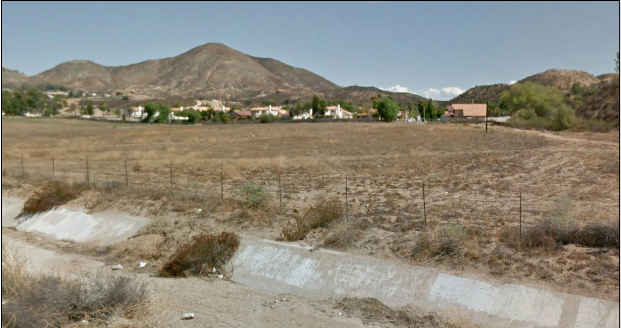
Figure 6. Proposed Bundy Canyon Basin, looking NE over the old alluvial fan,
