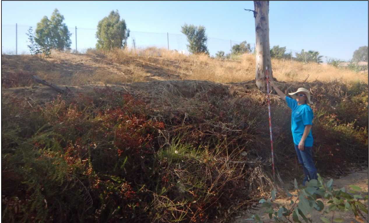
Figure 4. Approximately 20 feet of erosion in the Como Street stream channel.
